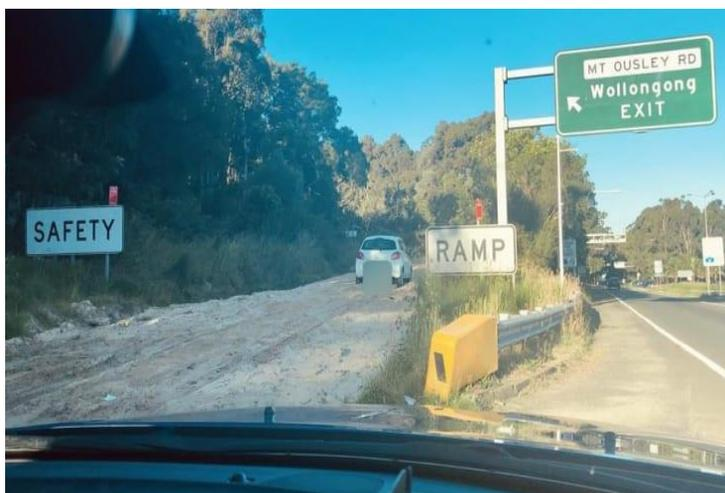
Truck 'arrestor beds' or 'sand traps' are designed to stop heavy vehicles at the bottom of steep hills if they run out of brakes.
